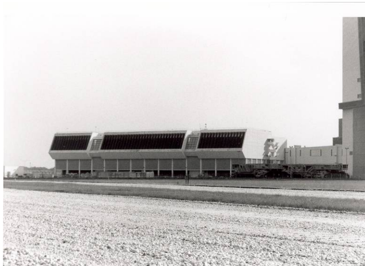
Photo 6.3. Launch Control Center, looking south. (Source: Archaeological Consultants, Inc., 1996)
