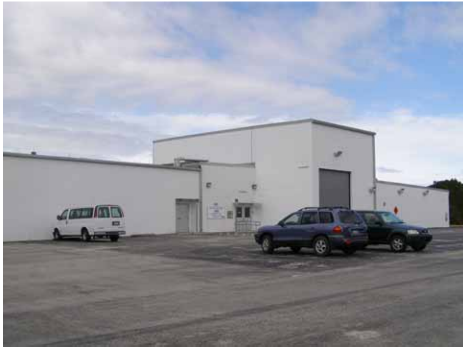
Photo 1. Parachute Refurbishment Facility, South elevation, camera facing northeast. (Source: Archaeological Consultants, Inc., 2007)
