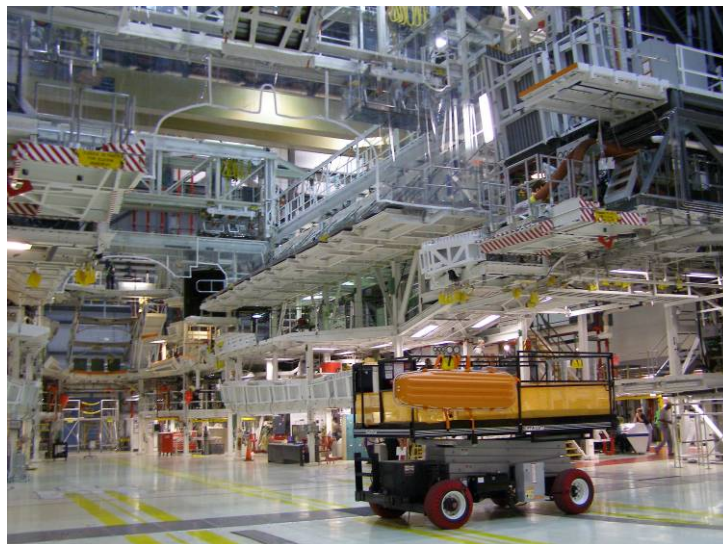
Photo 6.18. Orbiter Processing Facility High Bay 1 interior, looking southwest. (Source: Archaeological Consultants, Inc., 2006)
