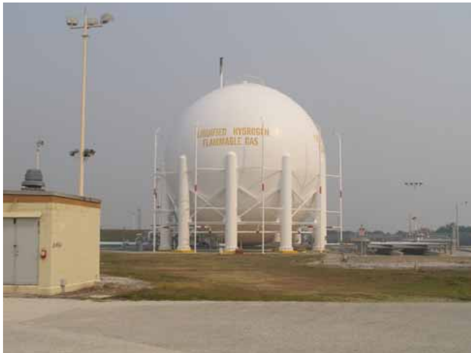
Photo 4. LC 39A, Liquid Hydrogen Facility, facing south. (Source: Archaeological Consultants, Inc., 2007)
