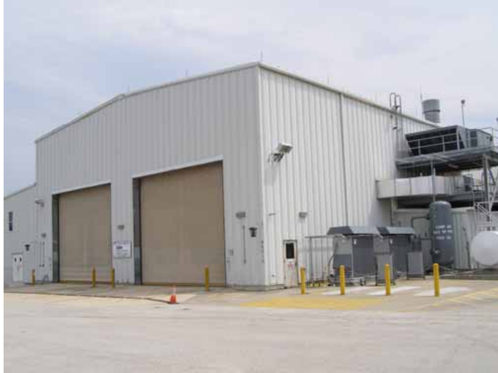
Photo 13. SRB Paint Building, north and east elevations. (Source: Archaeological Consultants, Inc., 2006)
