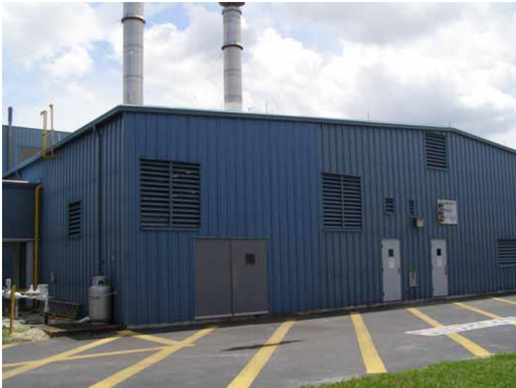
Photo 6. SRB ARF, chiller building. (Source: Archaeological Consultants, Inc., 2006)
