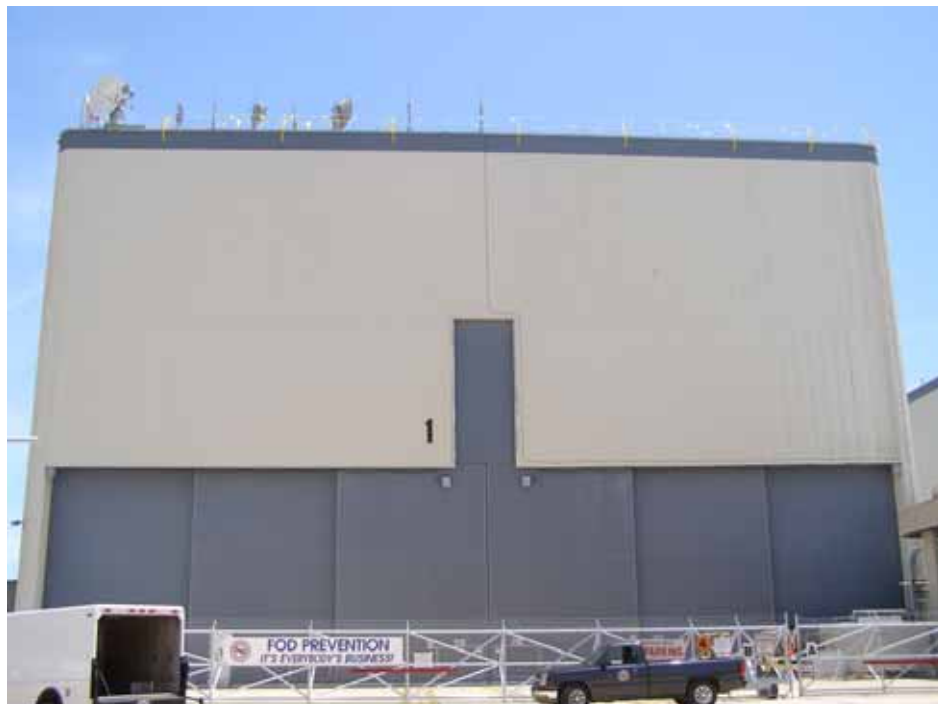
Photo 2. Orbiter Processing Facility High Bay 1, north elevation. (Source: Archaeological Consultants, Inc., 2006)
