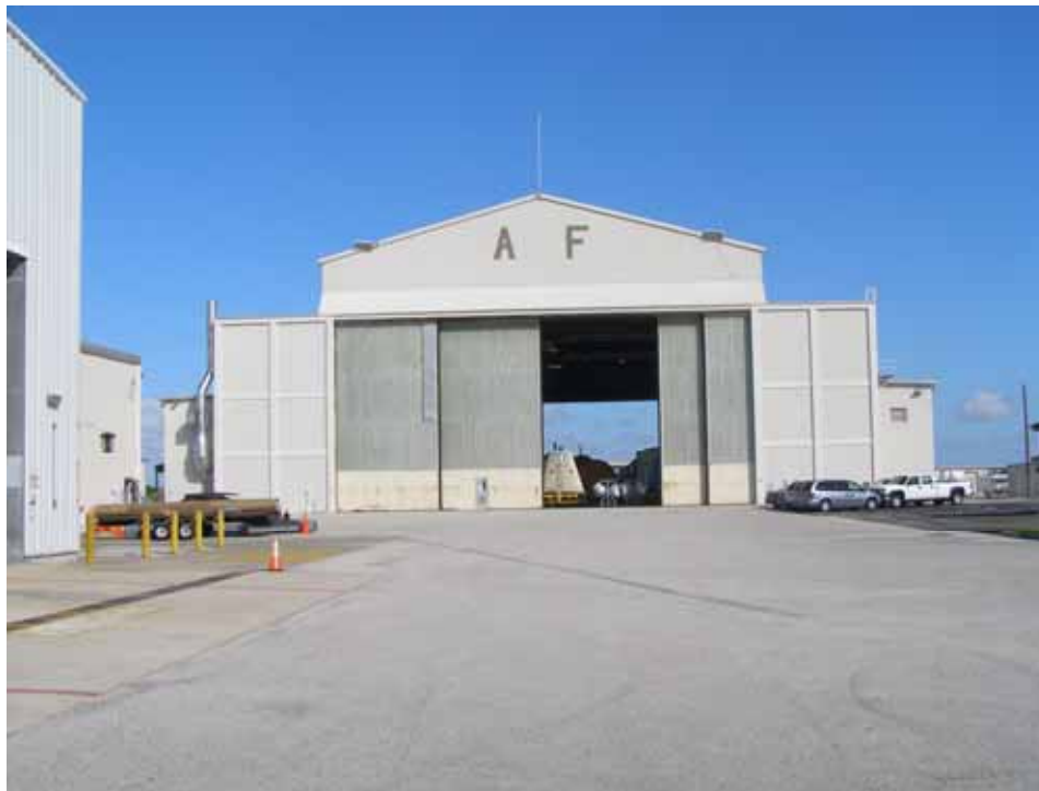
Photo 4. Hangar AF, east elevation. (Source: Archaeological Consultants, Inc., 2006)
