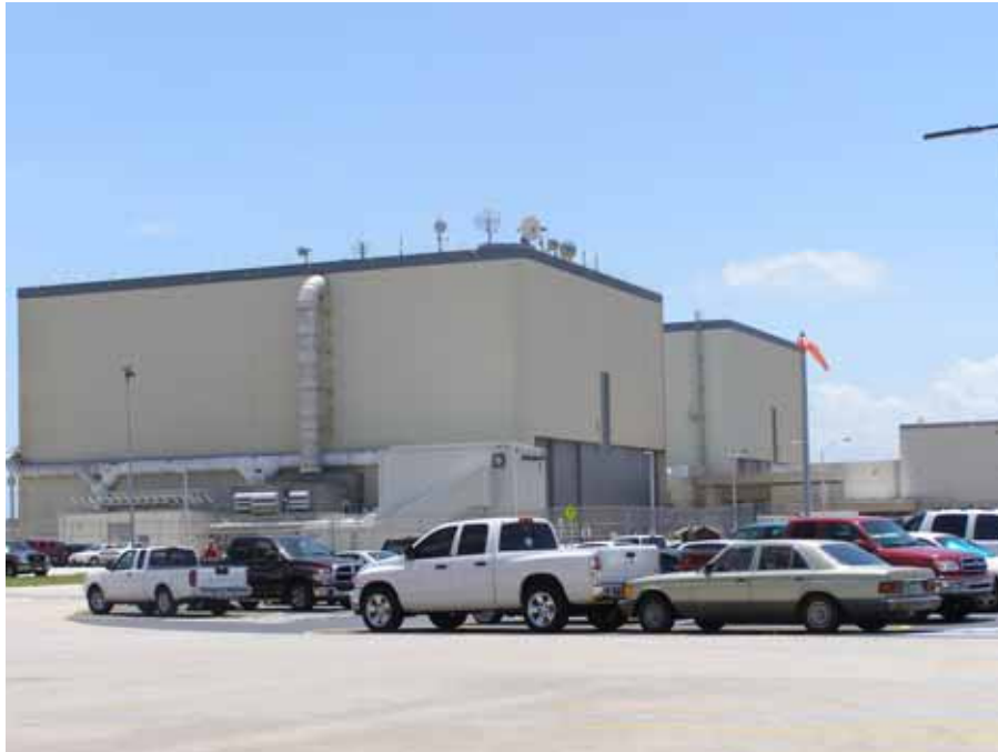
Photo 1. Orbiter Processing Facility, north and east elevations. (Source: Archaeological Consultants, Inc., 2006)
