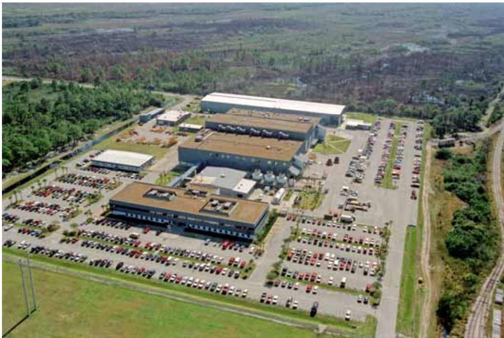
Photo 8. Aerial view of SRB Processing facility, 1996. (Source: NASA John F. Kennedy Space Center, KSC-396C-0968 FR36)
