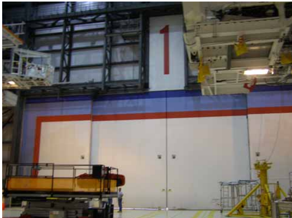
Photo 6. Orbiter Processing Facility High Bay 1, orbiter ingress/egress. (Source: Archaeological Consultants, Inc., 2006)
