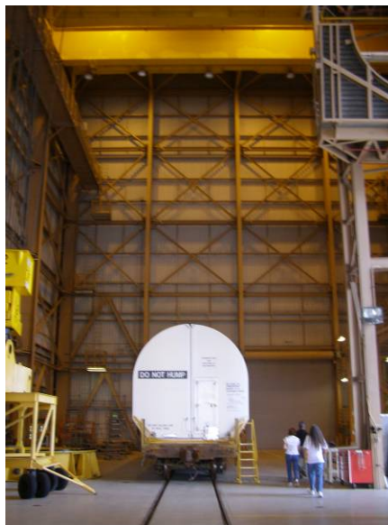
Photo 6.28. Rotation/Processing Building, interior looking west. (Source: Archaeological Consultants, Inc., 2006)
