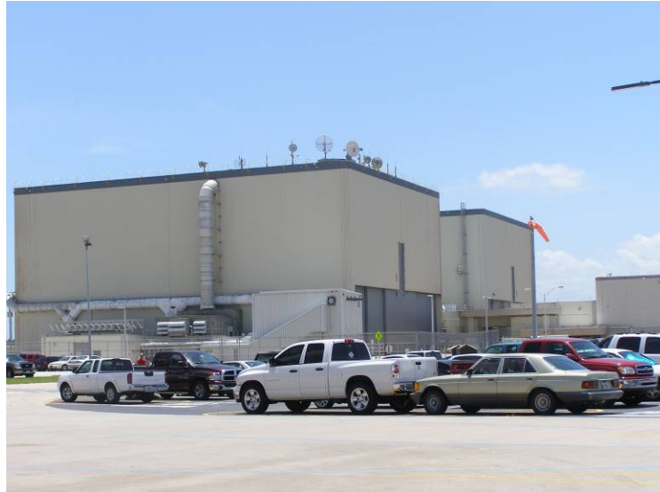
Photo 6.17. Orbiter Processing Facility (High Bays 1 and 2), north and east elevations. (Source: Archaeological Consultants, Inc., 2006)
