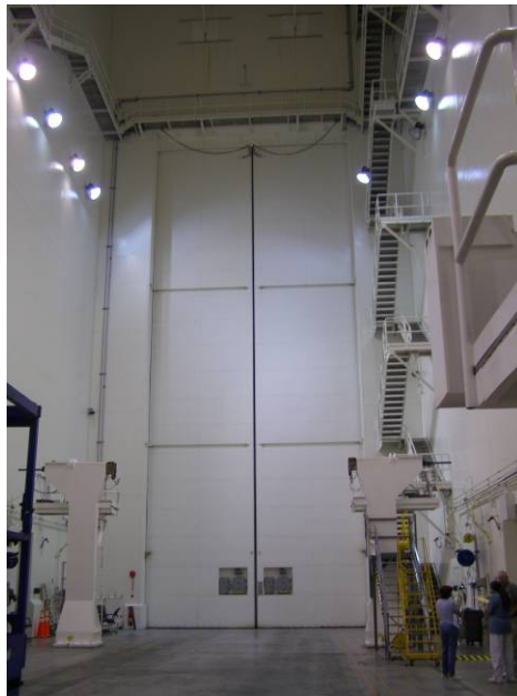
Photo 6.37. Canister Rotation Facility, clean room interior, looking east. (Source: Archaeological Consultants, Inc., 2006)
