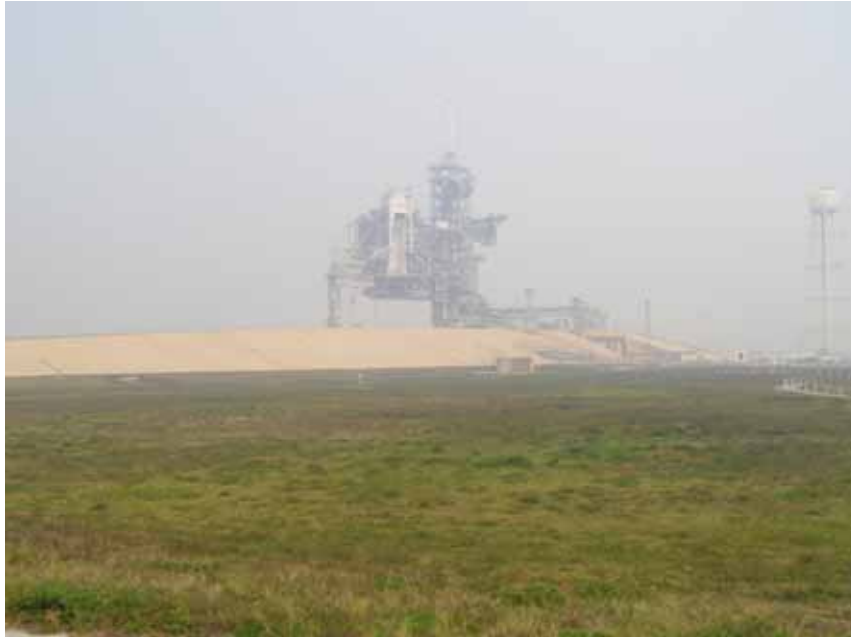
Photo 1. Launch Pad 39B, facing northwest. (Source: Archaeological Consultants, Inc., 2007)
