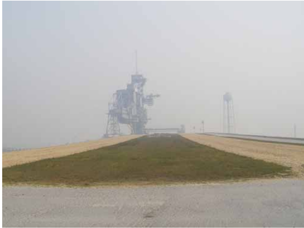
Photo 3. Crawlerway towards Launch Pad 39A, camera facing north. (Source: Archaeological Consultants, Inc., 2007)
