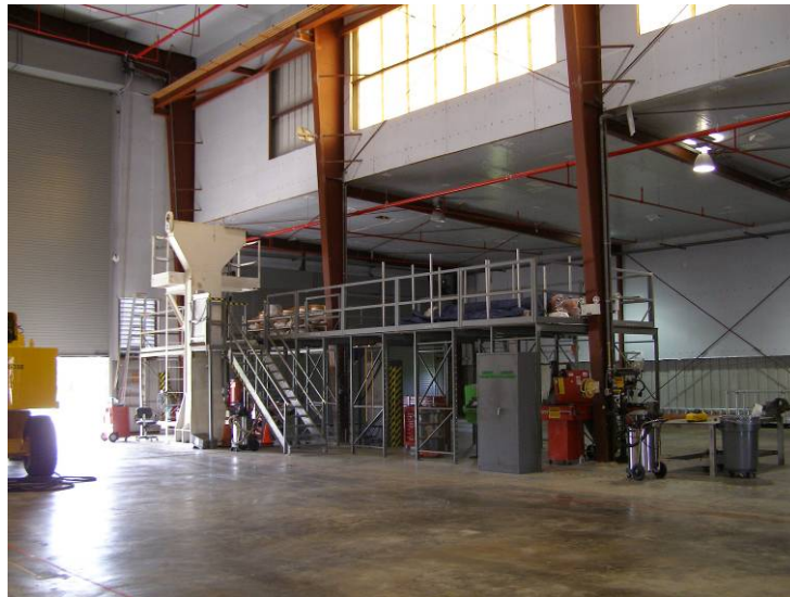
Photo 6.38. Canister Rotation Facility, interior to southeast. (Source: Archaeological Consultants, Inc., 2006)
