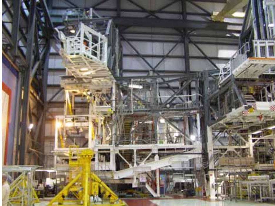
Photo 5. Orbiter Processing Facility High Bay 1, platform 513. (Source: Archaeological Consultants, Inc., 2006)
