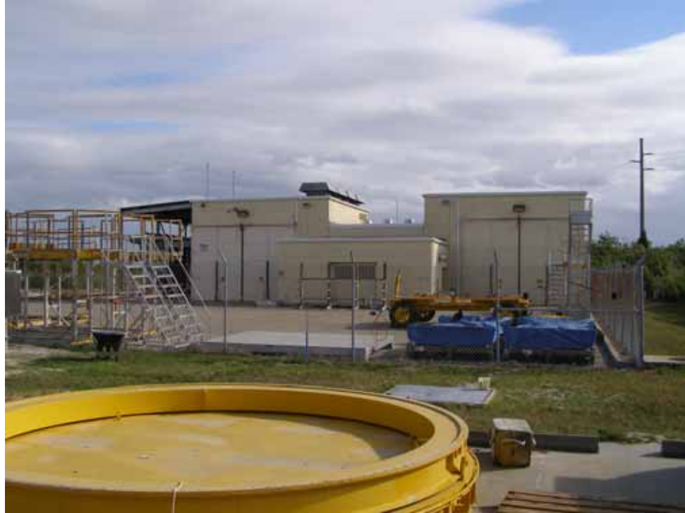
Photo 15. Multi-Media Blast Facility, north elevation. (Source: Archaeological Consultants, Inc., 2007)
