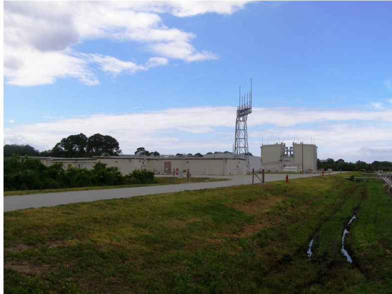
Photo 6.40. Hypergolic Maintenance and Checkout Area Historic District, looking northwest. (Source: Archaeological Consultants, Inc. 2007).
