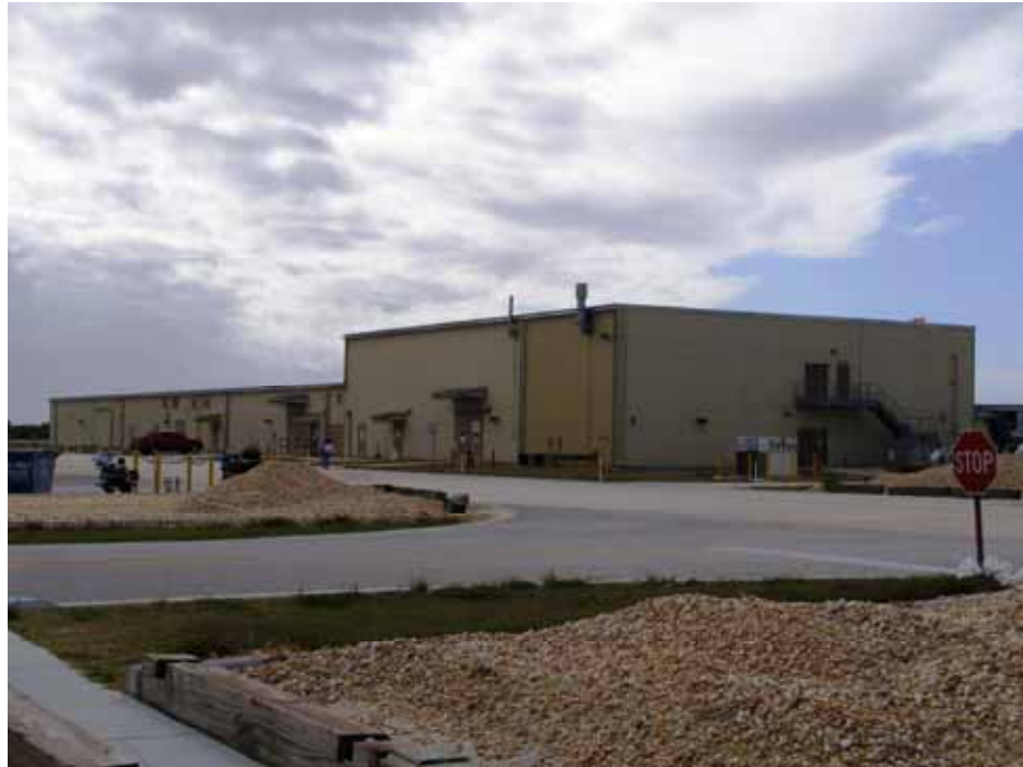
Photo 1. Thermal Protection System Facility, south and east elevations. (Source: Archaeological Consultants, Inc., 2007)
