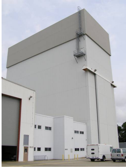
Photo 6.36. Canister Rotation Facility, south and east elevations. (Source: Archaeological Consultants, Inc., 2007)
