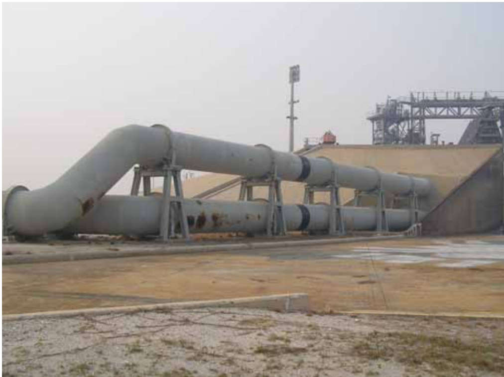
Photo 6. Launch Pad 39A, water suppression system, facing southeast. (Source: Archaeological Consultants, Inc., 2007)
