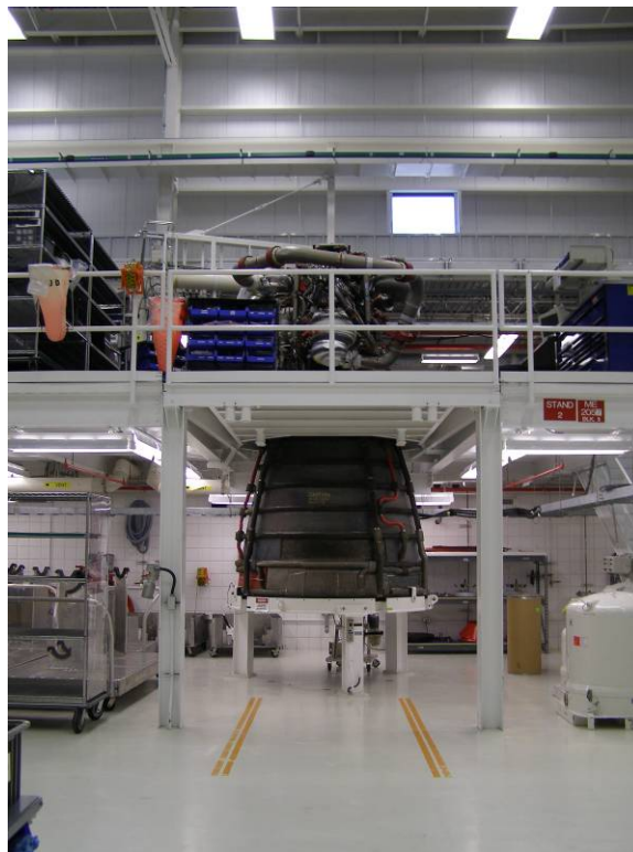
Photo 6.21. Space Shuttle Main Engine Facility at OPF High Bay 3, vertical stand. (Source: Archaeological Consultants, Inc., 2006)
