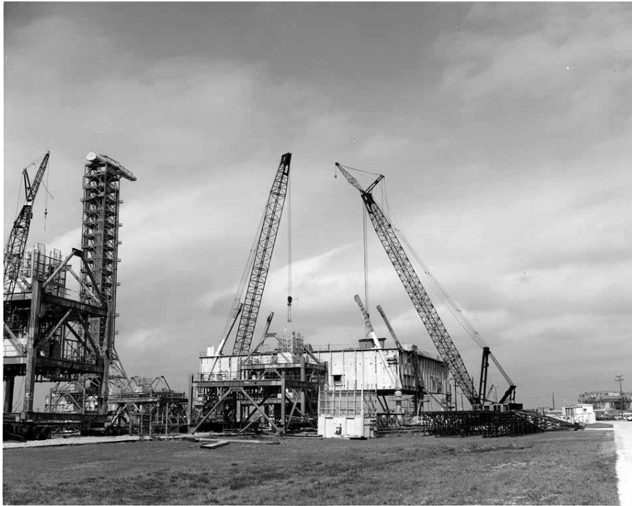
Photo 3. MLP during renovations for Space Shuttle Program, 1976. (Source: NASA John F. Kennedy Space Center, KSC-76C-0904)
