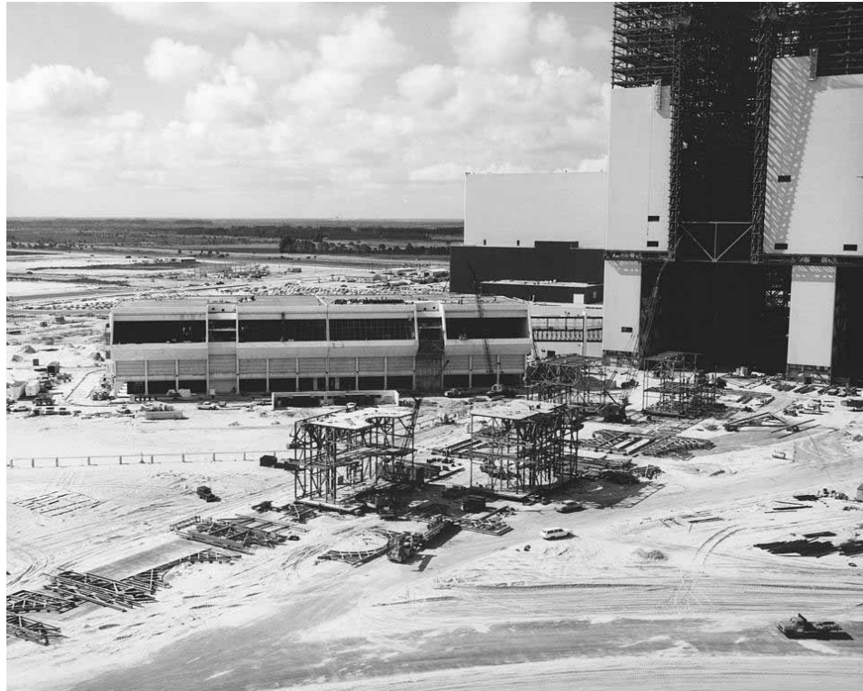
Photo 3. Aerial view of LCC construction, 1965. (Source: NASA John F. Kennedy Space Center, 65C-0990)
