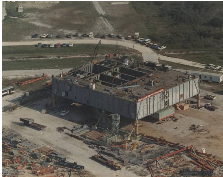
Photo 6.46. MLP modifications, September 1976. (Source: NASA Kennedy Space Center, KSC-76C-2754)
