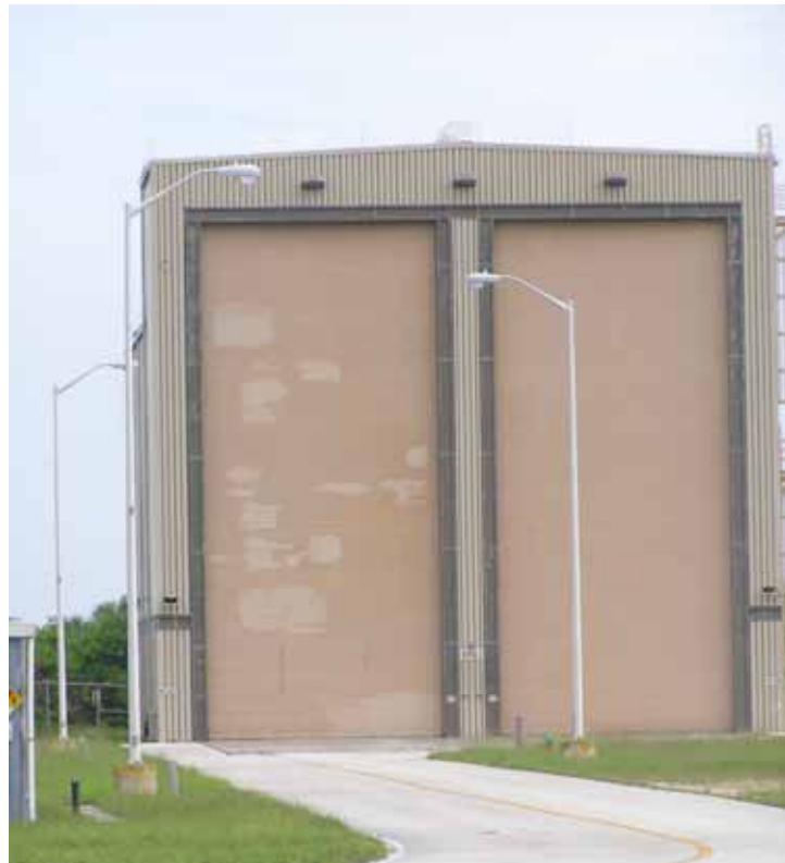
Photo 8. RPSF, Surge #2, south elevation. (Source: Archaeological Consultants, Inc., 2006)
