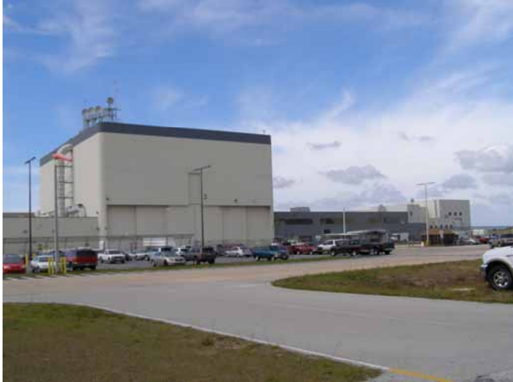
Photo 3. Orbiter Processing Historic District, OPF-3, camera facing northeast. (Source: Archaeological Consultants, Inc., 2007)
