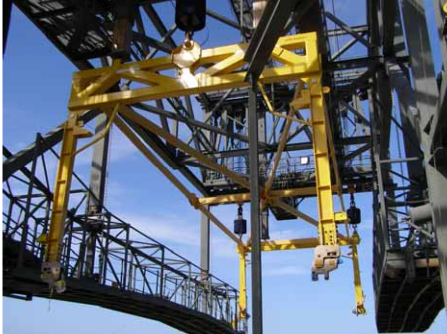
Photo 3. Mate-Demate Device, moveable platforms and slingback. (Source: Archaeological Consultants, Inc., 2006)
