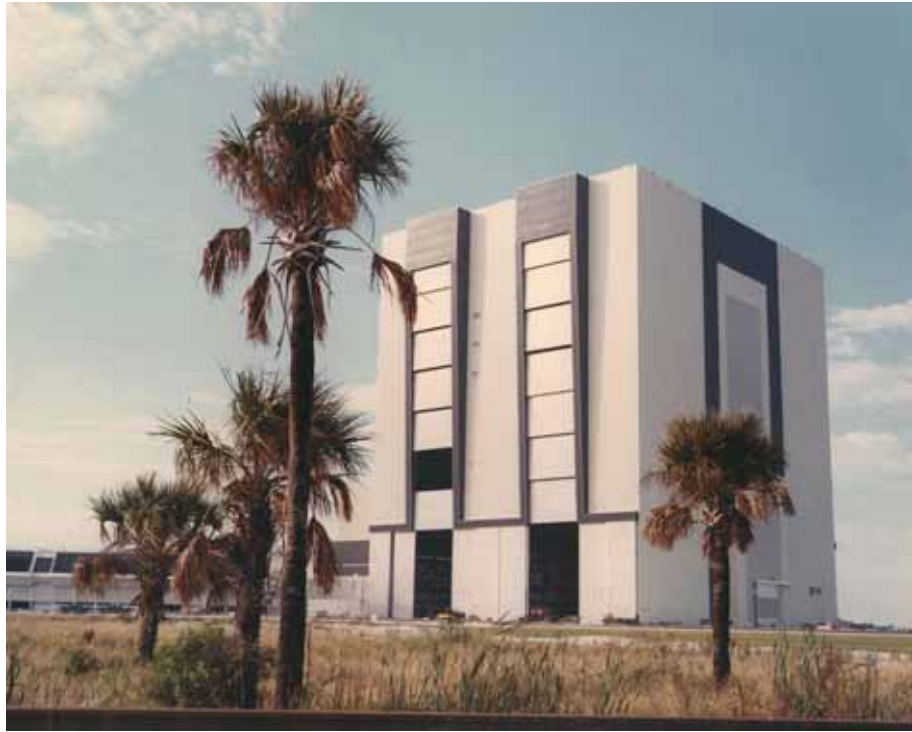
Photo 7. VAB upon completion, 1966. (Source: NASA John F. Kennedy Space Center, 66C-0525)
