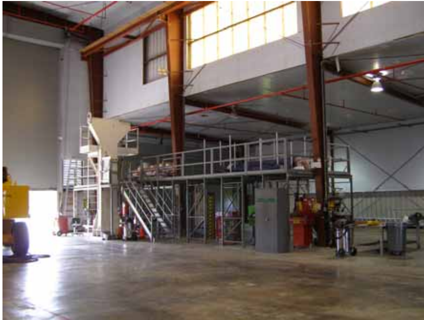
Photo 5. Canister Rotation Facility, interior to southeast. (Source: Archaeological Consultants, Inc., 2006)
