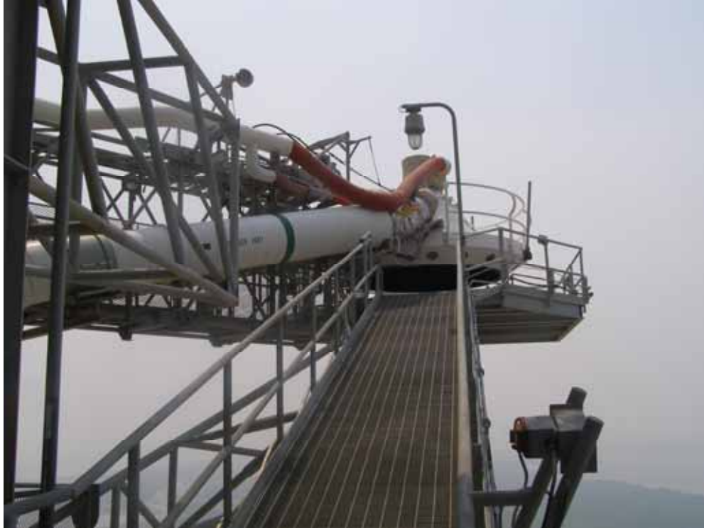
Photo 3. Launch Pad 39B, ET gaseous oxygen vent arm, facing east. (Source: Archaeological Consultants, Inc., 2007)
