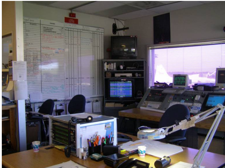
Photo 6.14. Landing Aids Control Building, control room looking southwest. (Source: Archaeological Consultants, Inc., 2006)
