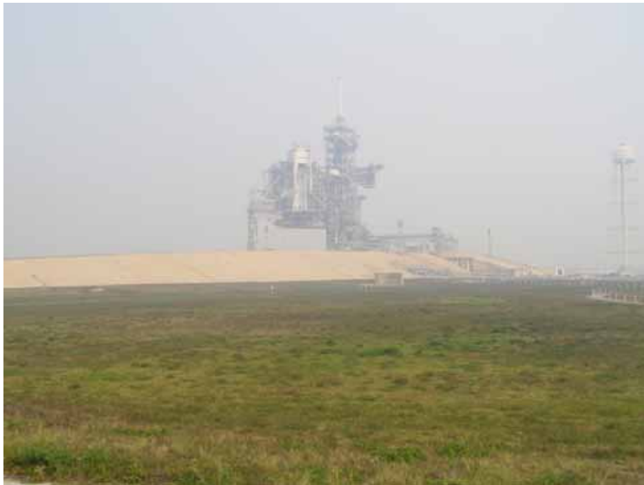
Photo 2. Launch Pad 39B, facing northwest. (Source: Archaeological Consultants, Inc., 2007)
