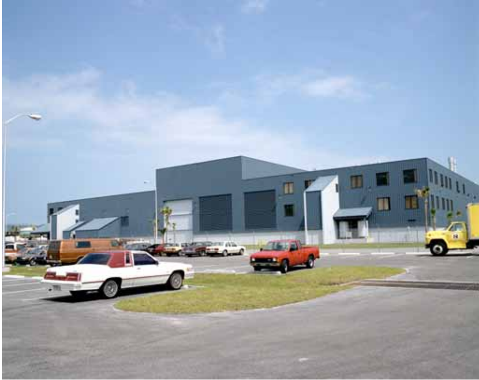
Photo 7. SRB Processing facility, 1987. (Source: NASA John F. Kennedy Space Center, KSC-387C-566 FR02)
