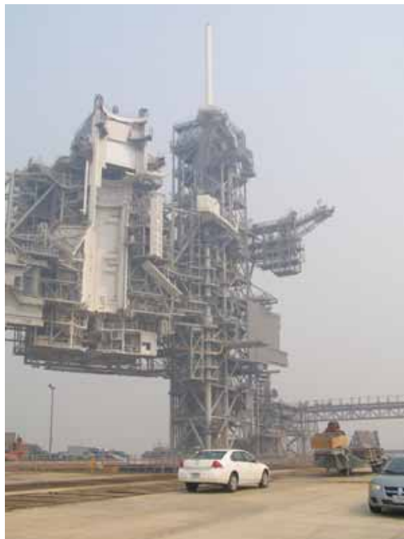
Photo 2. Launch Pad 39A, FSS, facing northwest. (Source: Archaeological Consultants, Inc., 2007)
