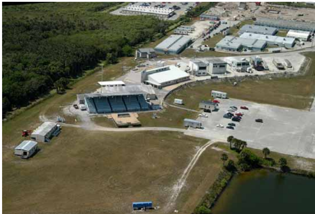
Photo 2. Aerial view of Press Site, 2004. (Source: NASA John F. Kennedy Space Center, KSC-04PD-0915)
