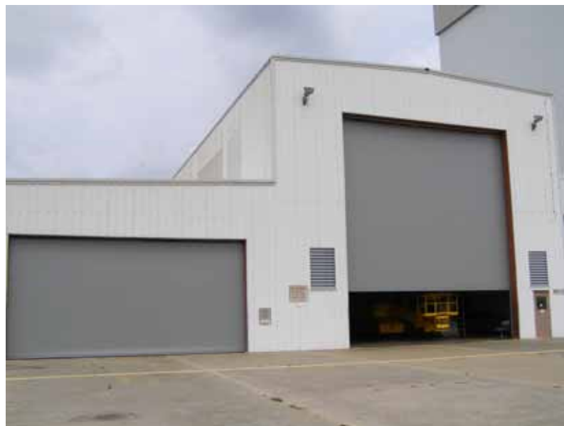
Photo 2. Canister Rotation Facility, east elevation. (Source: Archaeological Consultants, Inc., 2006)
