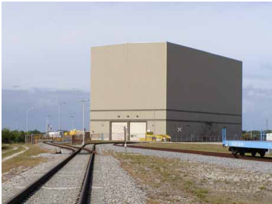
Photo 2. Rotation/Processing Building, west and south elevations. (Source: Archaeological Consultants, Inc., 2007)
