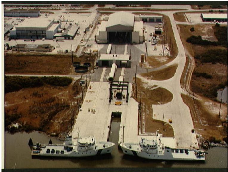
Photo 6.25. Aerial view of the SRB Disassembly and Refurbishment Complex, July 1981. (Source: NASA Johnson Space Center, S81-33609)
