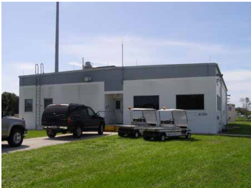
Photo 2. Landing Aids Control Building, north elevation. (Source: Archaeological Consultants, Inc., 2006)
