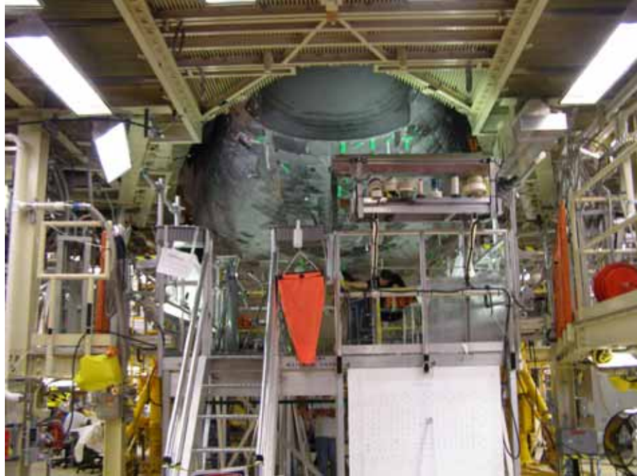
Photo 3. Orbiter Processing Facility High Bay 3, orbiter nose and platforms, looking south. (Source: Archaeological Consultants, Inc., 2006)
