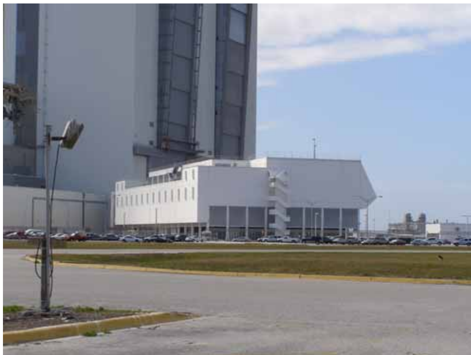
Photo 2. Launch Control Center, south and east elevations, camera facing northwest. (Source: Archaeological Consultants, Inc., 2007)
