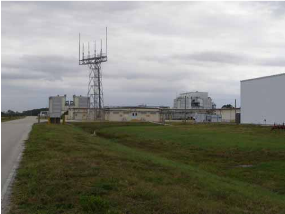
Photo 3. Hypergol Support Building, north elevation, camera facing southwest.. (Source: Archaeological Consultants, Inc., 2007)
