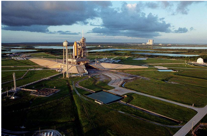
Photo 6.8. Aerial view of Space Shuttle Discovery at LC 39A, 2000. (Source: NASA John F. Kennedy Space Center, KSC-00PP-1297)
