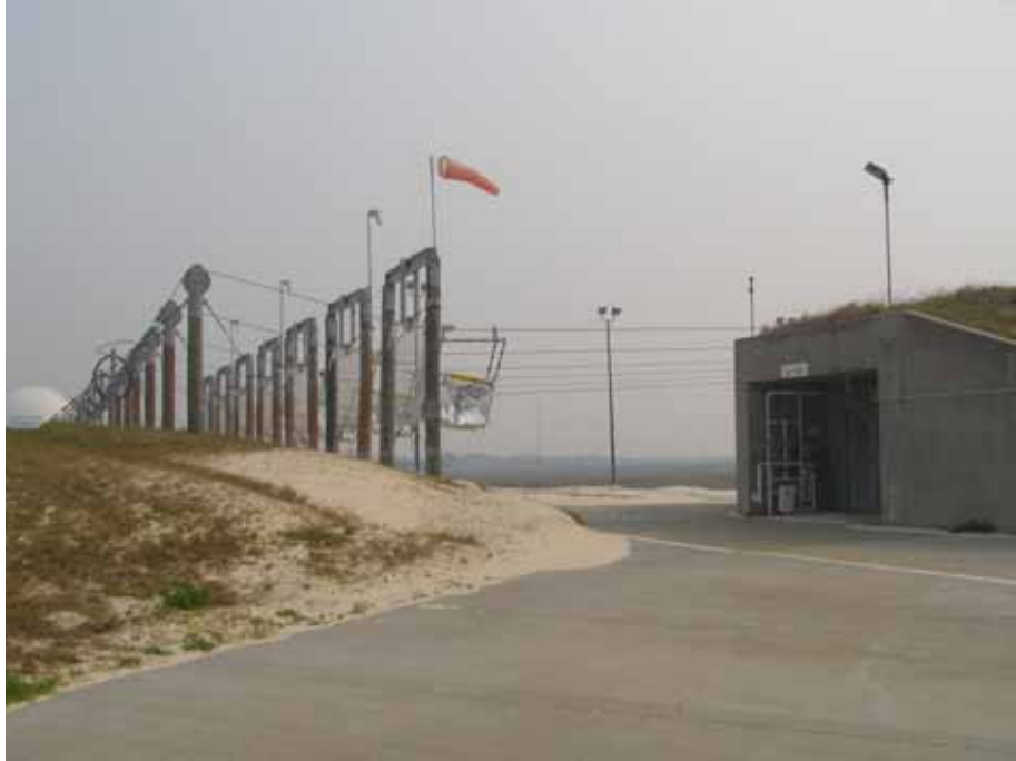
Photo 5. LC 39A, Slidewire Termination Facility, facing southeast. (Source: Archaeological Consultants, Inc., 2007)
