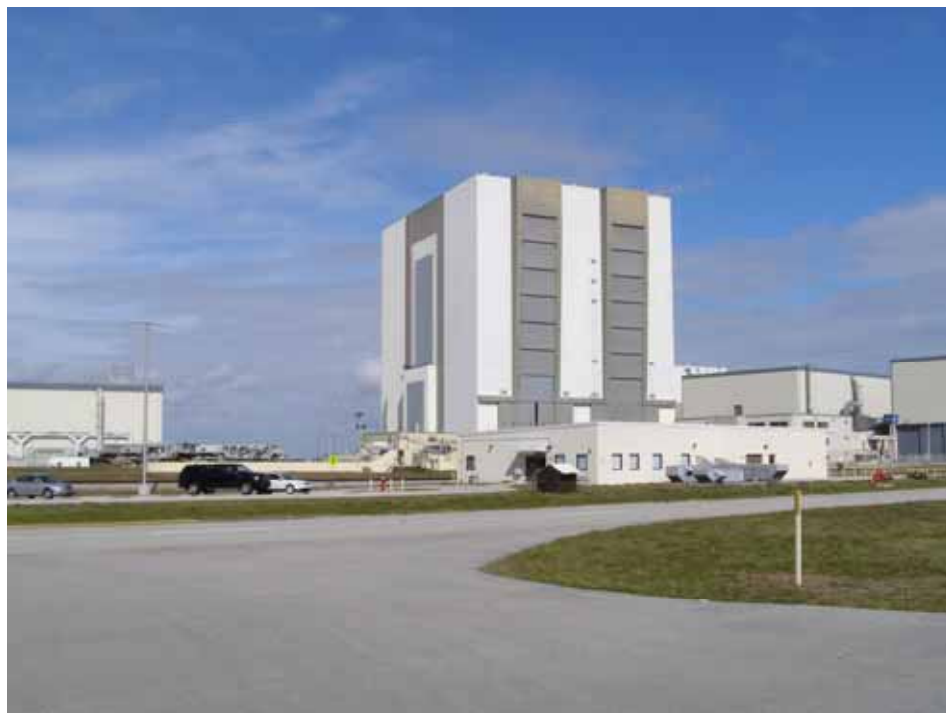
Photo 2. Vehicle Assembly Building, north and west elevations. (Source: Archaeological Consultants, Inc., 2007)
