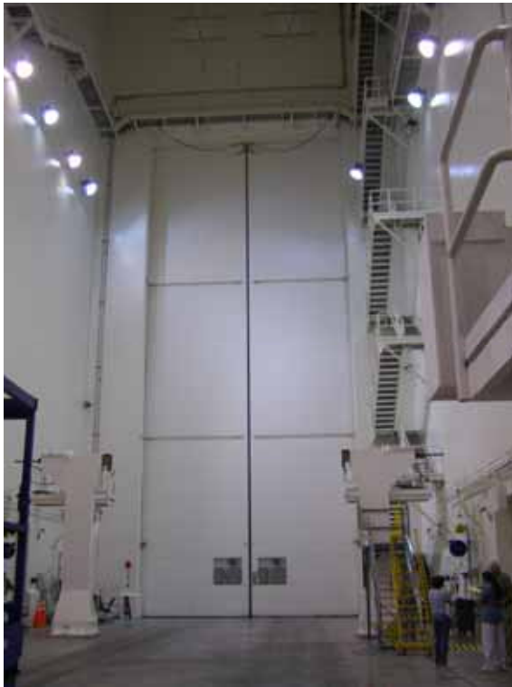
Photo 4. Canister Rotation Facility, clean room interior looking east. (Source: Archaeological Consultants, Inc., 2006)
