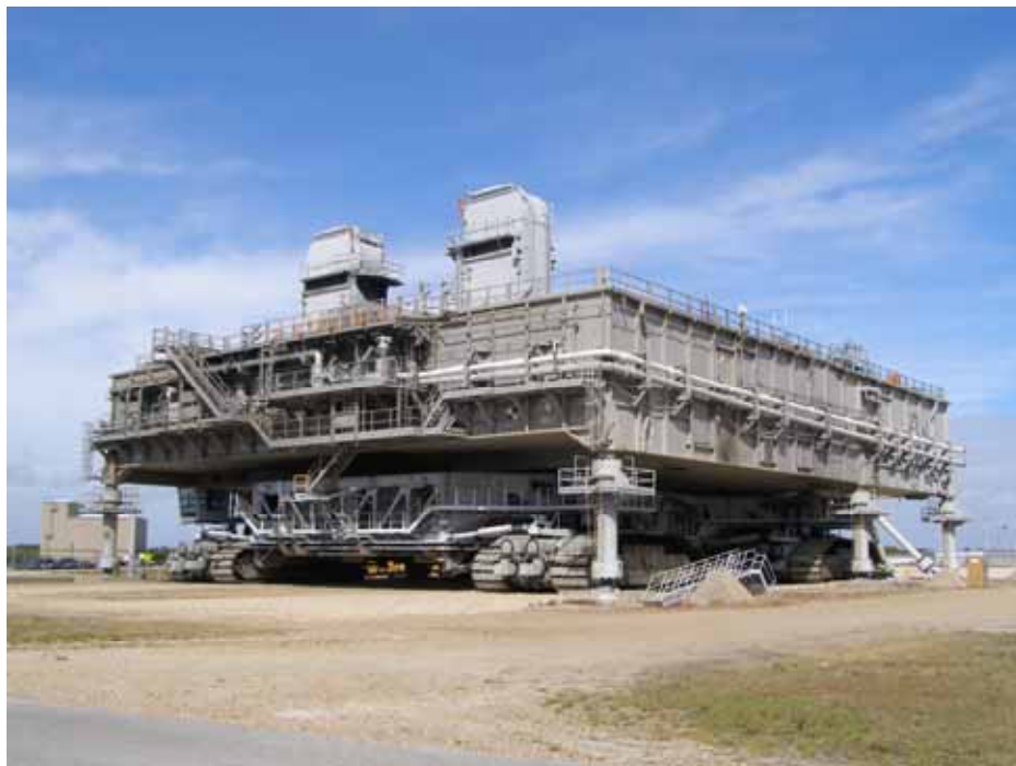
Photo 2. Crawler with MLP, Sides 2 and 3 (Source: Archaeological Consultants, Inc., 2007)
