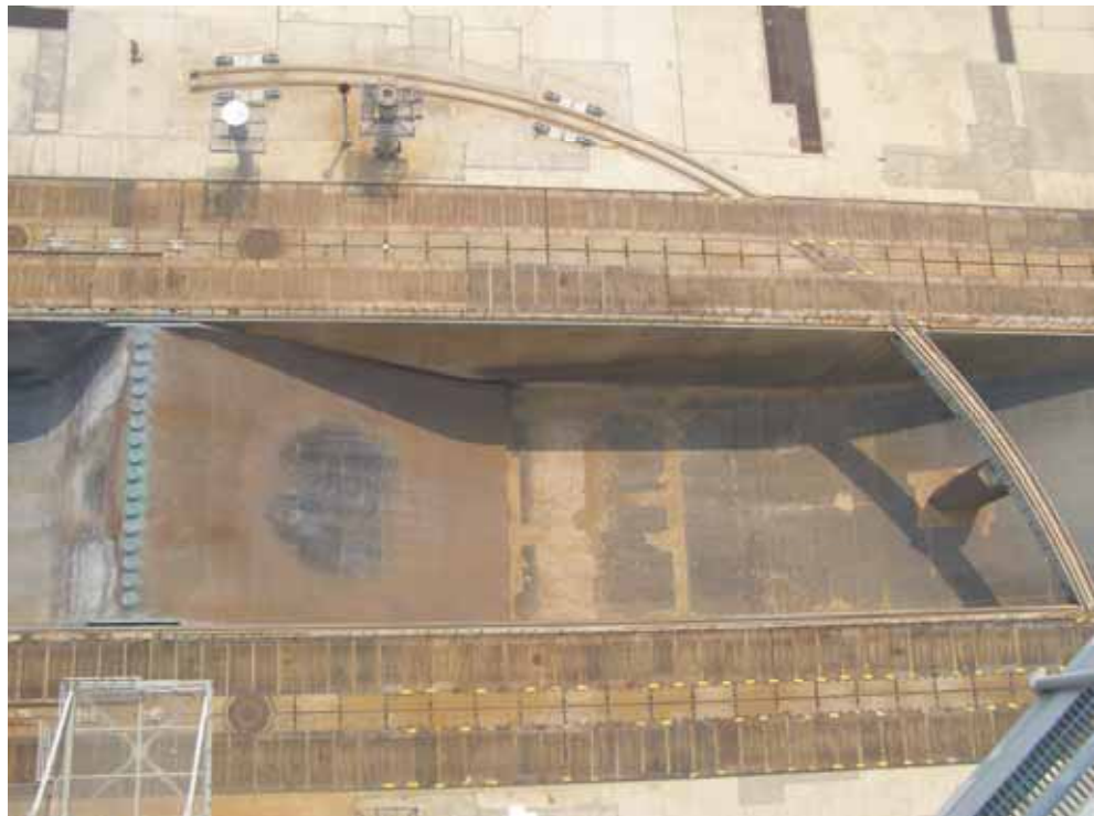
Photo 4. Launch Pad 39B, Flame Trench deflector and rail track for RSS, facing east. (Source: Archaeological Consultants, Inc., 2007)
