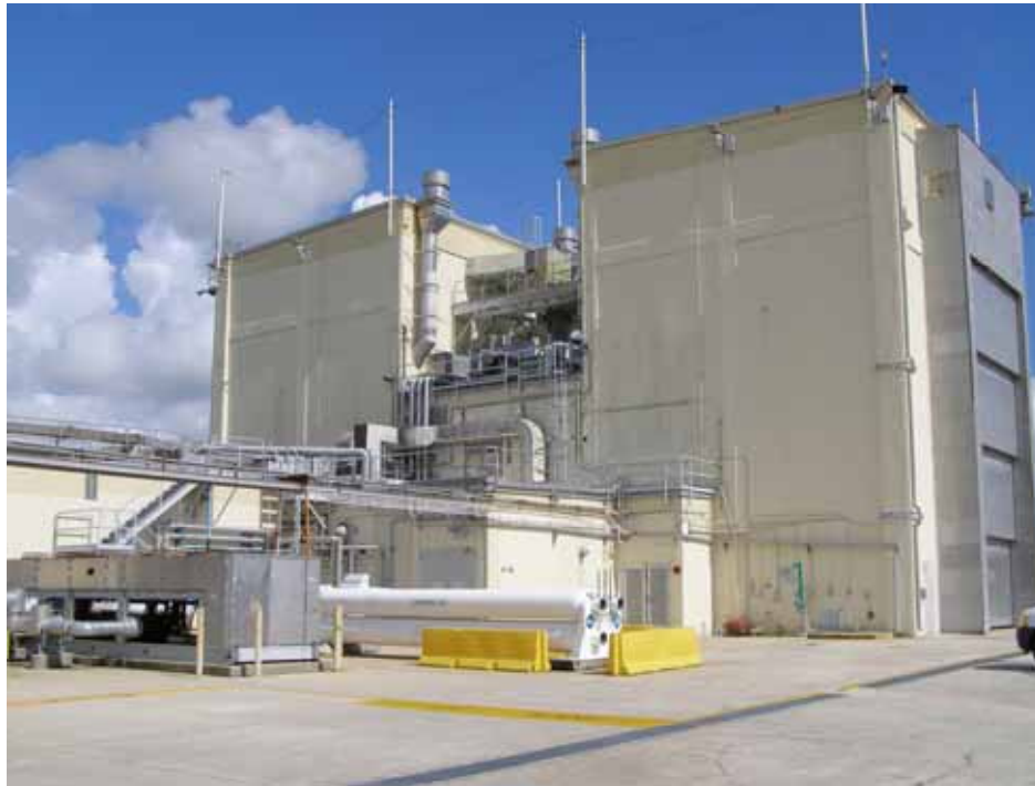
Photo 2. HMP (North) facility, south elevation. (Source: Archaeological Consultants, Inc., 2006)
