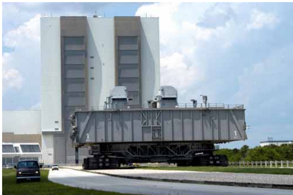
Photo 6. MLP atop Crawler Transporter, 2003. (Source: NASA John F. Kennedy Space Center, KSC-03PD-2357)
