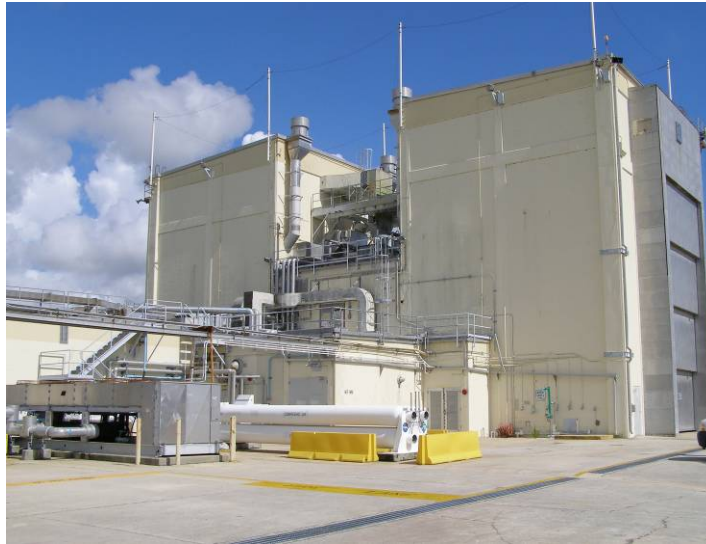
Photo 6.41. Hypergol Module Processing (North) Facility, south elevation. (Source: Archaeological Consultants, Inc., 2006)
