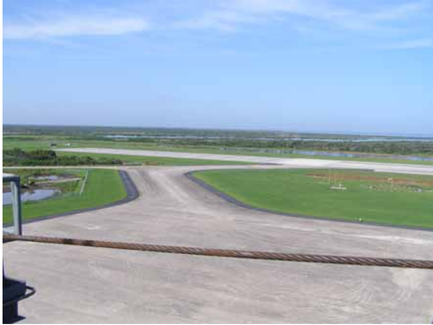
Photo 3. Shuttle Landing Facility (Runway), looking southwest. (Source: Archaeological Consultants, Inc., 2006)
