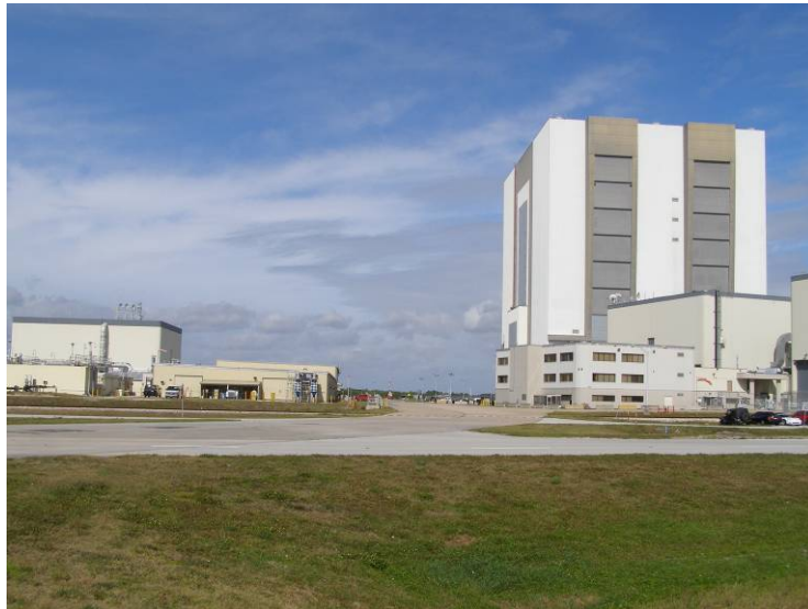
Photo 6.16. Orbiter Processing Facilities, looking east. (Source: Archaeological Consultants, Inc., 2007)
