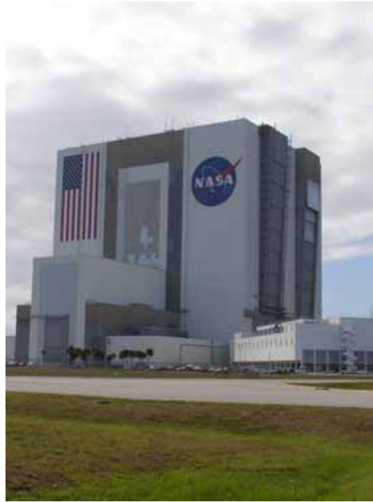
Photo 1. Vehicle Assembly Building, south and east elevations. (Source: Archaeological Consultants, Inc., 2007)
