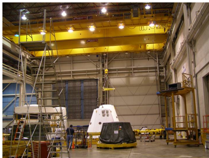
Photo 6.31. SRB ARF Manufacturing Building, lifting crane. (Source: Archaeological Consultants, Inc., 2006)
