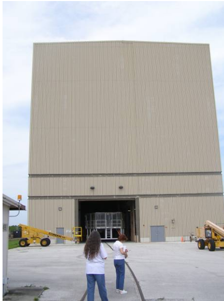
Photo 6.27. Rotation/Processing Building, east elevation. (Source: Archaeological Consultants, Inc., 2006)
