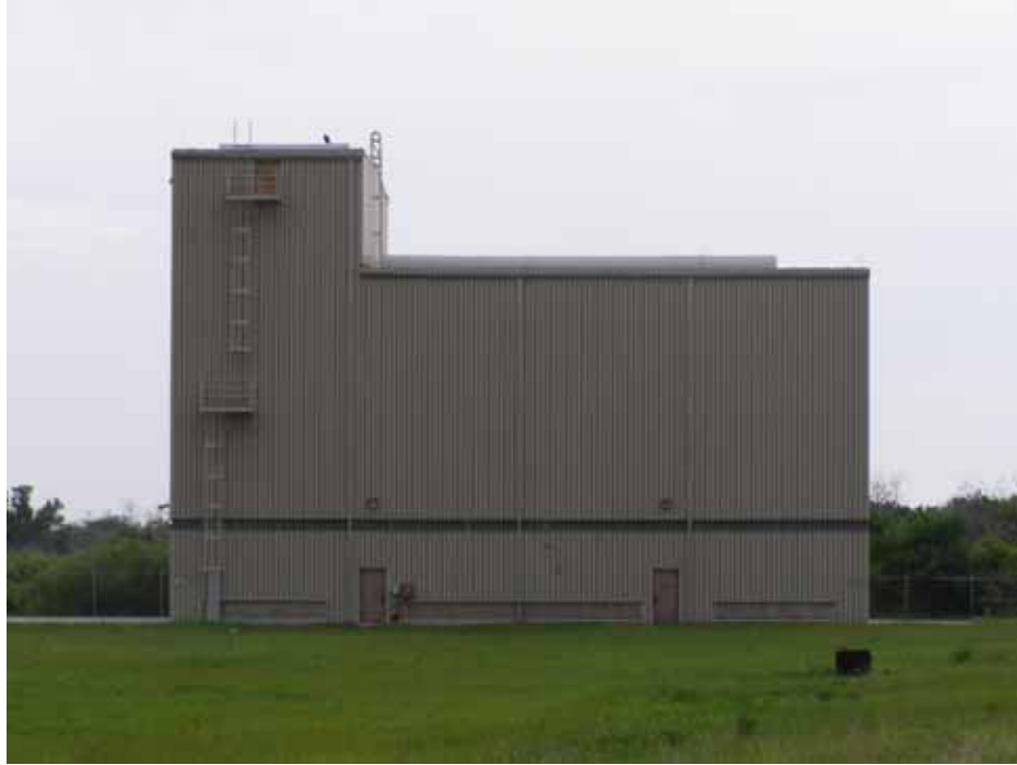
Photo 7. RPSF, Surge #1, west elevation. (Source: Archaeological Consultants, Inc., 2006)
