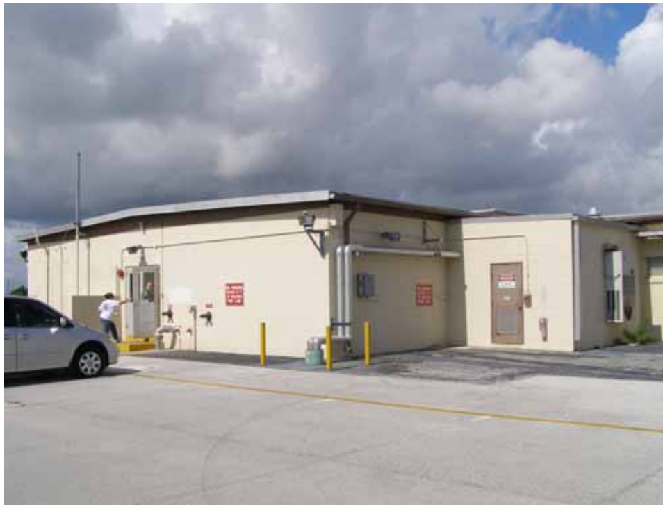
Photo 4. Hypergol Support Building, south elevation. (Source: Archaeological Consultants, Inc., 2006)
