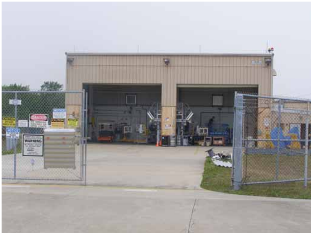
Photo 14. Thrust Vector Control Deservicing Building, south elevation. (Source: Archaeological Consultants, Inc., 2007)
