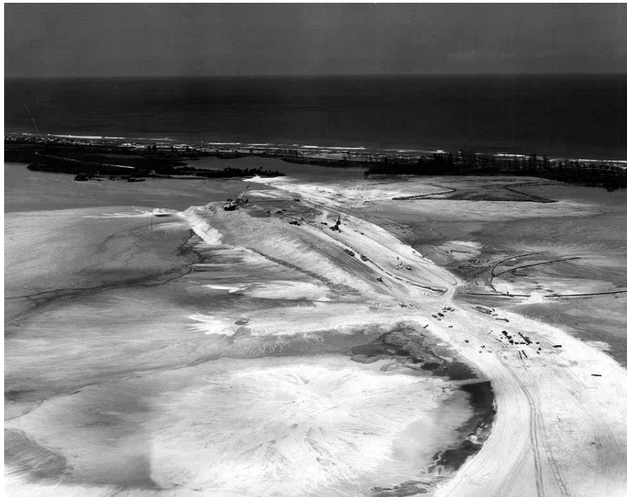
Photo 6. Aerial view of Launch Complex 39A construction, 1963. (Source: NASA John F. Kennedy Space Center, LOC63-5654)
