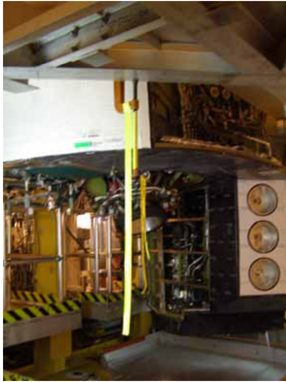
Photo 3. Platform Level 1, HMP (North), looking northeast. (Source: Archaeological Consultants, Inc., 2006)
