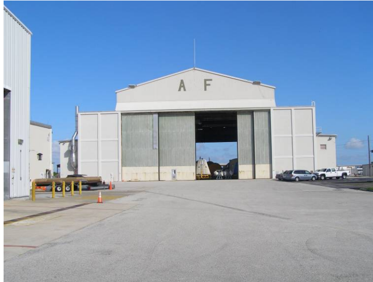
Photo 6.26. Hangar AF, east elevation. (Source: Archaeological Consultants, Inc., 2006)
