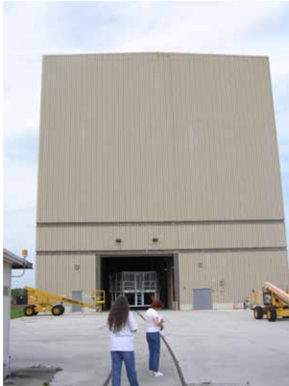
Photo 1. Rotation/Processing Building, east elevation. (Source: Archaeological Consultants, Inc., 2006)
