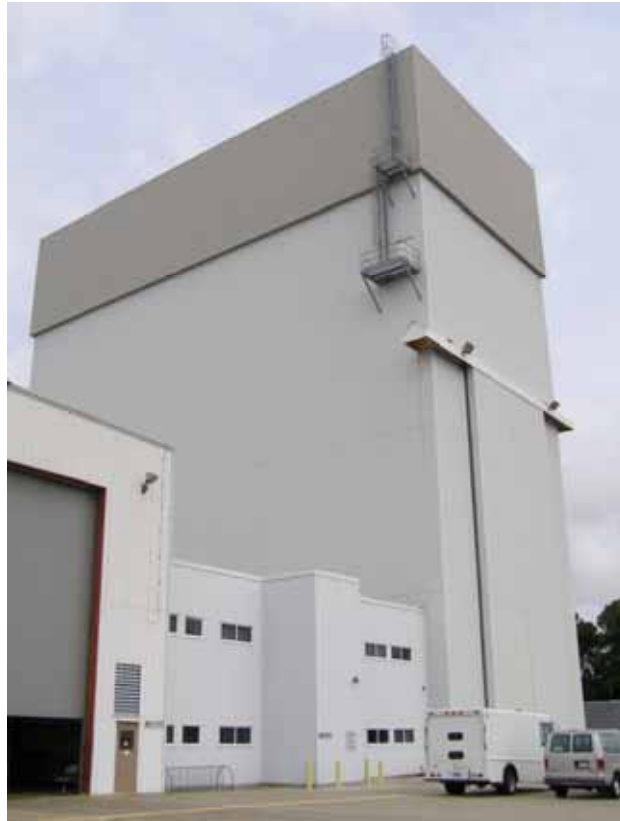
Photo 1. Canister Rotation Facility, south and east elevations. (Source: Archaeological Consultants, Inc., 2006)
