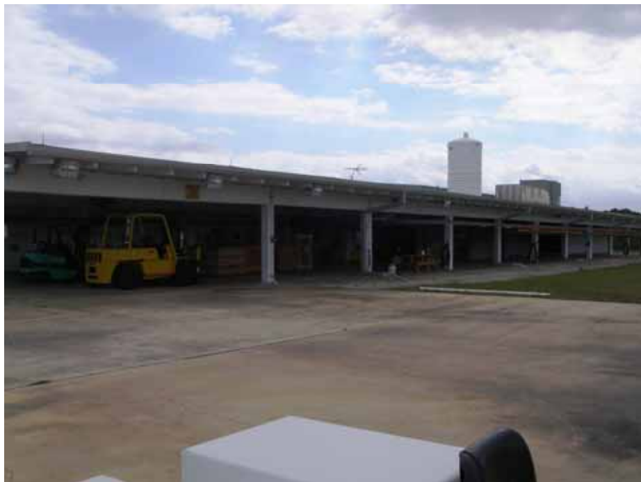
Photo 2. Parachute Refurbishment Facility, north elevation, camera facing southwest. (Source: Archaeological Consultants, Inc., 2007)
