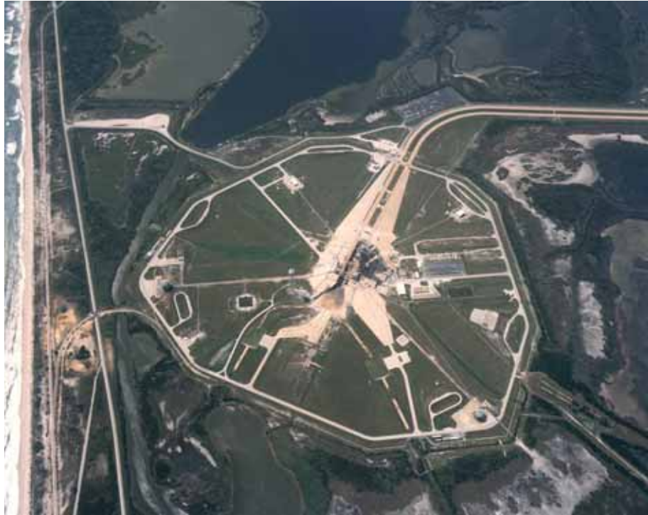
Photo 1. Aerial view of LC39A, 1984. (Source: NASA John F. Kennedy Space Center, KSC-384C-3061 FR08)
