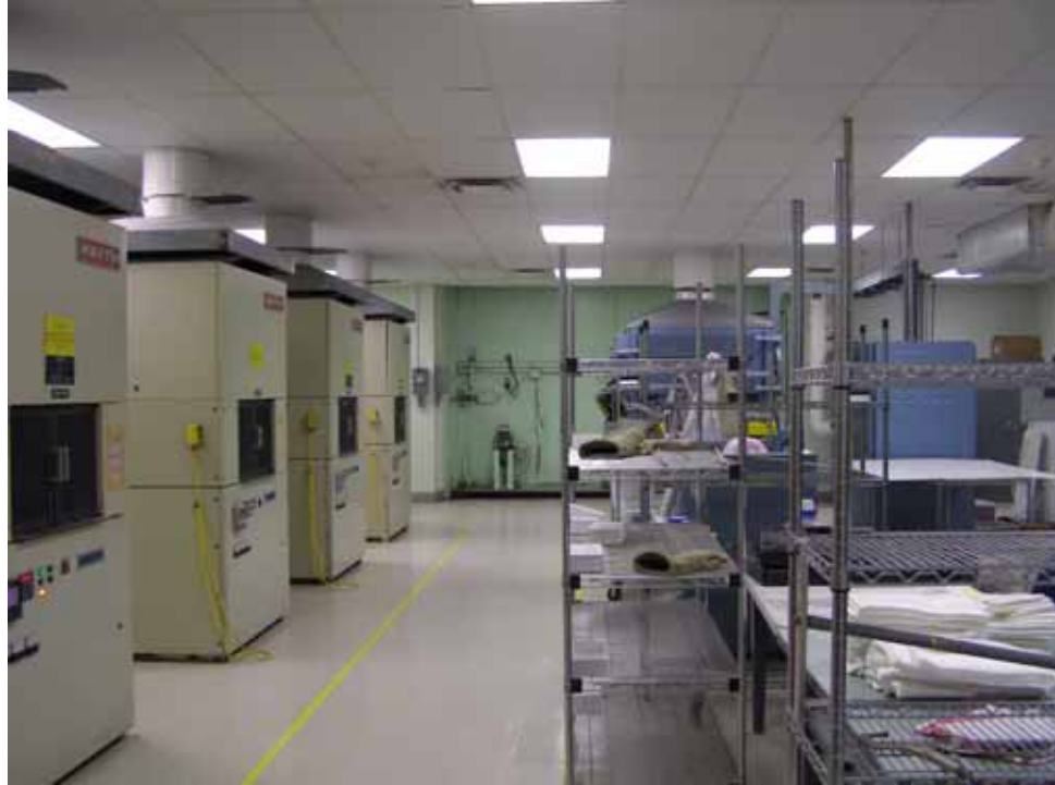
Photo 5. Thermal Protection System Facility, heat cleaning room. (Source: Archaeological Consultants, Inc., 2006)
